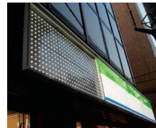
This photo shows the underlying layer of white LEDs (at the left) used in a FamilyMart store-façade sign
