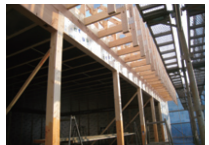
Building using the frame-and-panel method (viewed from the entrance)
