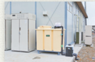
A water storage tank was installed outside as mains supplies had not yet been restored.
