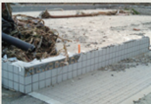
All that was left of the store after the tsunami was the foundation.
