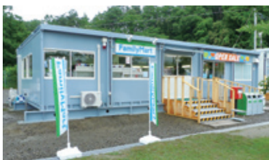
Unit-type prefabrication enables temporary stores to be built in a short time.
