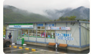
Prefabricated unit store
