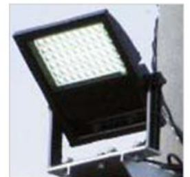
LED parking lot lighting
