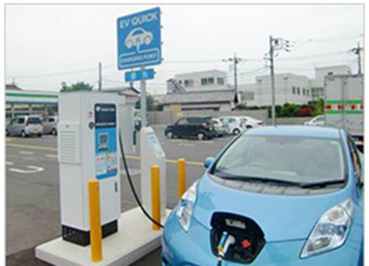
Installation of electric vehicle quick chargers
